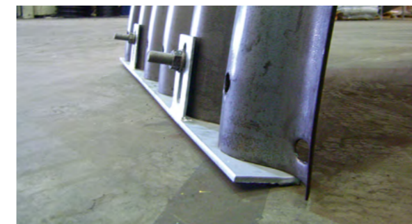
Fot. 1. Flat steel attached to the structure with an open cross-section
